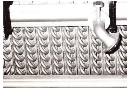
Figure 3.3.1 Non Condensing super heater
